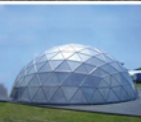
Geodesic Dome Roof
