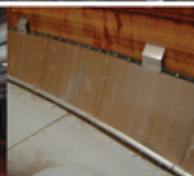
Floating Roof Seal
